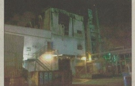
TUAS PLANT: Technicians at the Eco SWM waste management plant were transporting an oblong into a funnel leading to an incinerator when the fire broke out early yesterday morning.
